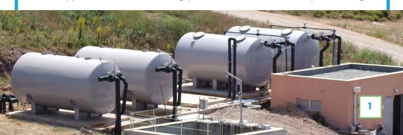
mineral deposit. During this backwash procedure, suspended solid materials and other particles kept in the mineral deposit are discharged from the backwash line of the filter. After backwash procedure, filters start to operate in service position again.
